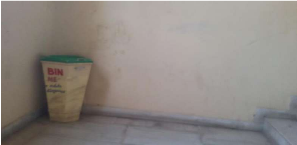
Dust bins at every floor steps
