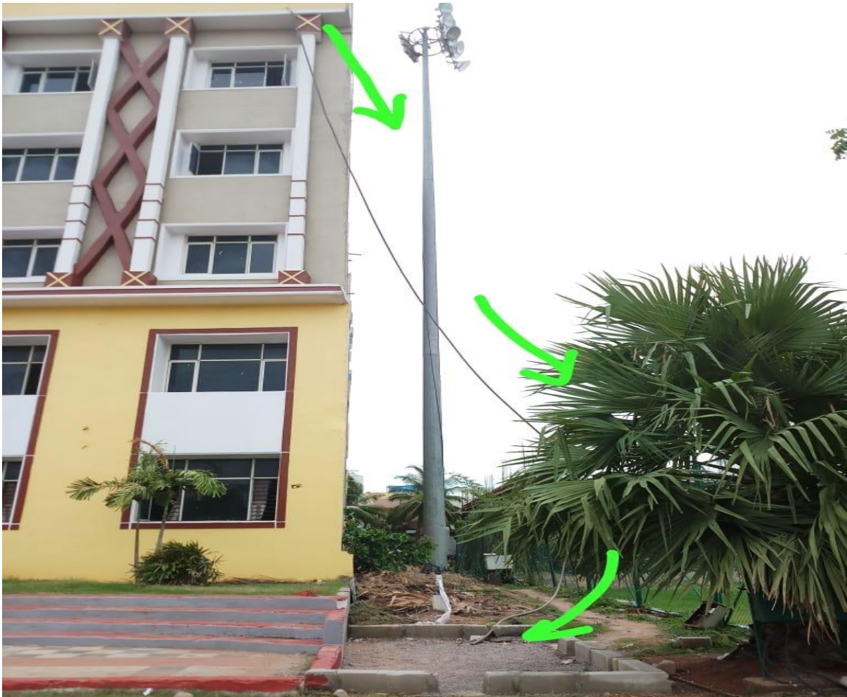
Rain Water storage pits below the building
