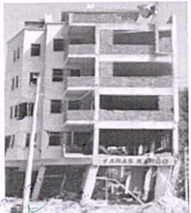
Fig. 2 Failure of stilt floor during earthquakes
